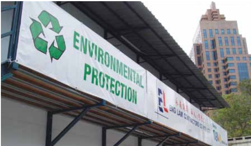
Safety banner at our construction site.
