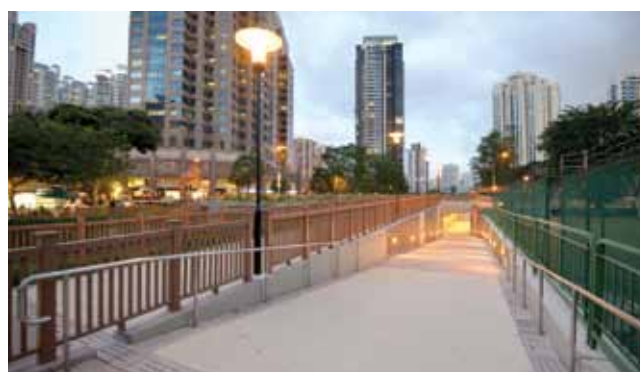
Alexander Canal is one of OKP's completed projects during the year.
