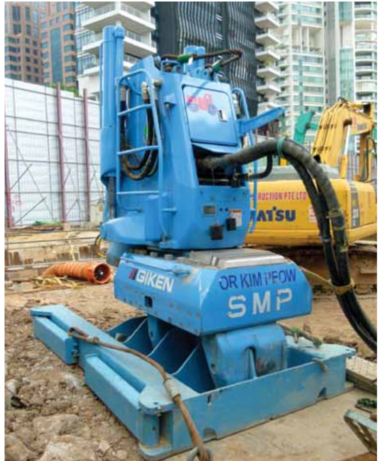
Newly purchased silent piler being used at our worksite.
