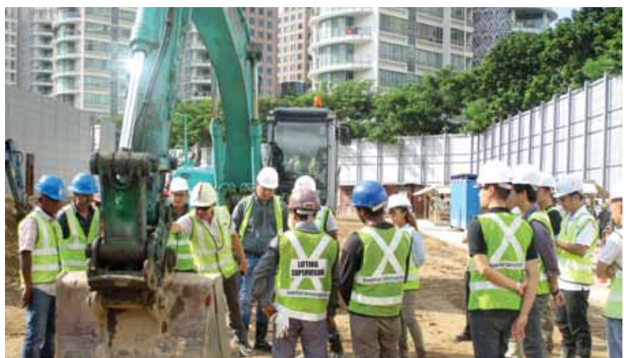
Group inspection of an excavator at a worksite.
