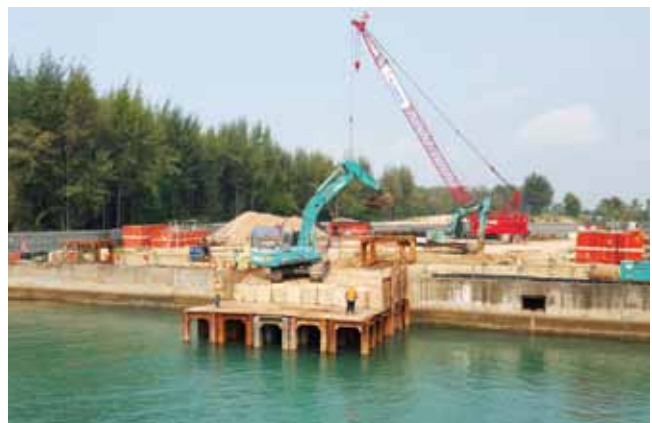
OKP is involved in the widening of Tanah Merah Coast Road.
