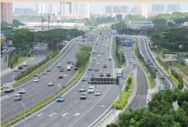
OKP's largest public sector project to date involved the widening of the CTE from PIE to Braddell Interchange.
