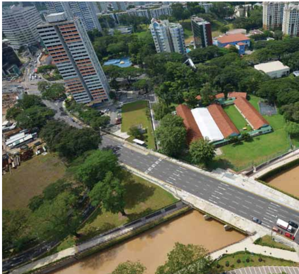
Alexander Canal is one of OKP's completed construction projects during the year.
