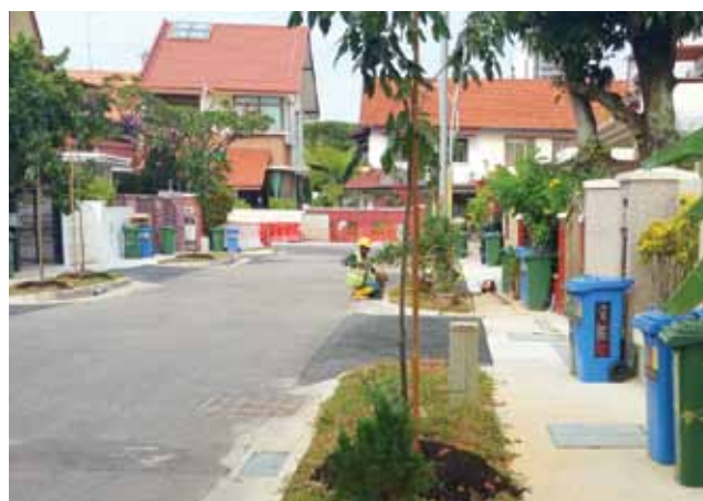
Improvement to roadside drains in Geylang is one of OKP's completed maintenance projects in 2015.
