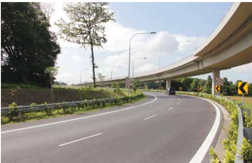
OKP completed the expansion of the CTR/TPE/SLE Interchange in 2015.
