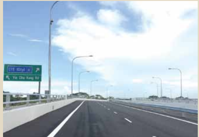
Expansion of CTE/TPE/SLE Interchange is one of OKP's completed construction projects in 2015.
