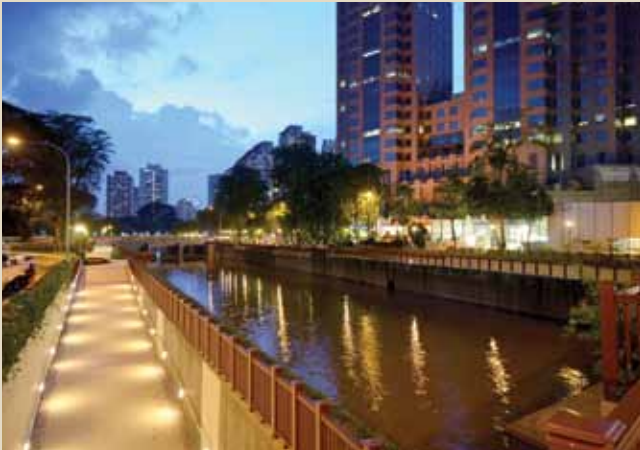
Alexander Canal is one of OKP's completed construction projects in 2015.
