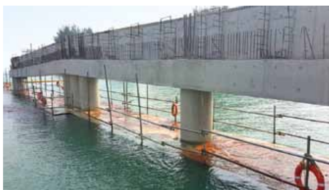
OKP is involved in the widening of Tanah Merah Coast Road.
