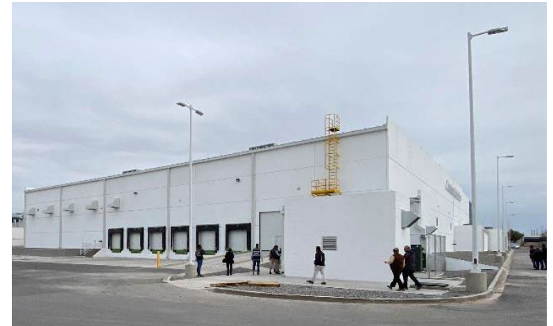
Warehouse, Dock and Label Printing Room
