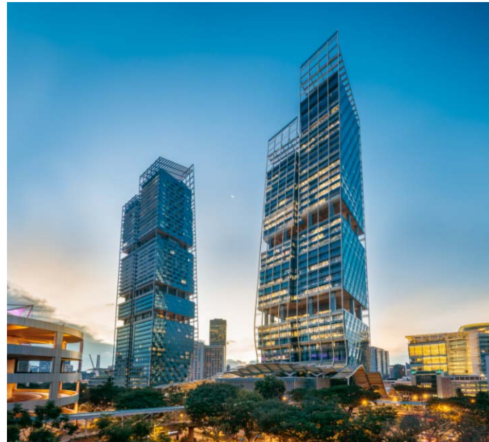
South Beach Tower
