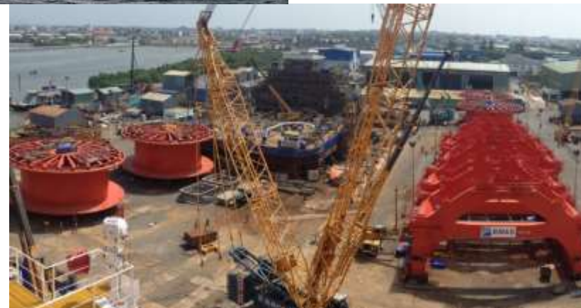
Reels & Cradles fabricated at TRIYARDS SOFEL in Vung Tau, Vietnam
