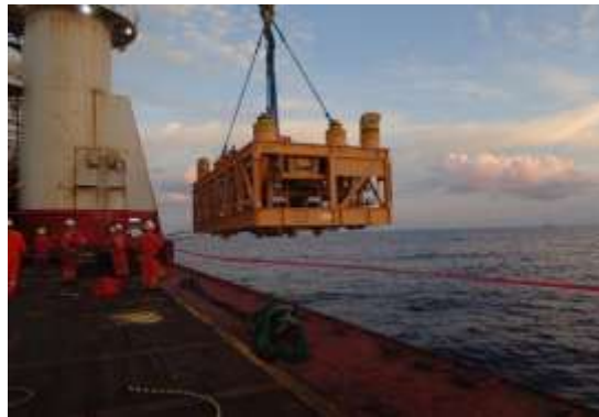
Manifold installation
