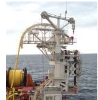
Flexible flowline installation
