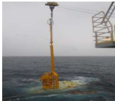
Transfer PLEM to lay tower
