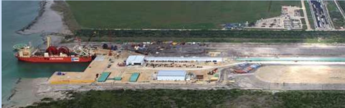
Deepwater spool base, marine support and fabrication facility
