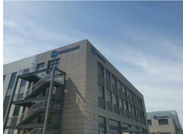
Plant Extension in Changzhou, China
