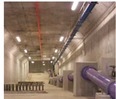
▲ Common Service Tunnel
