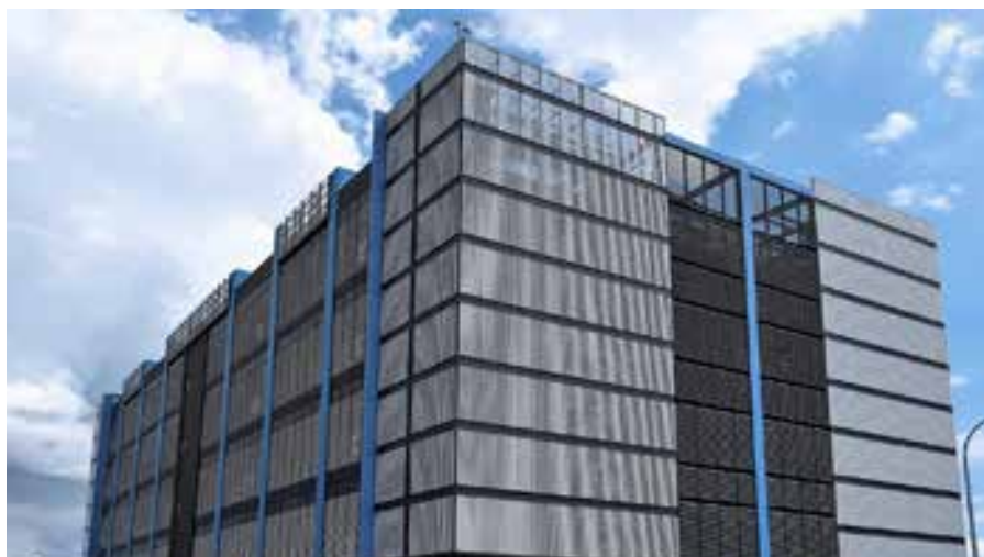
Launched in December 2020, the StarHub Hyperscale Data Centre @ Loyang located in the AirTrunk SGP1 campus provides flexibility, interconnected ecosystem, one-stop managed services and power efficiency.
