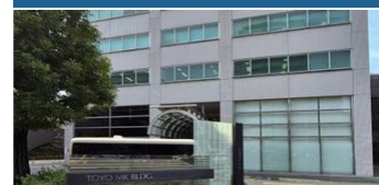
Toyo MK Fuso Building
