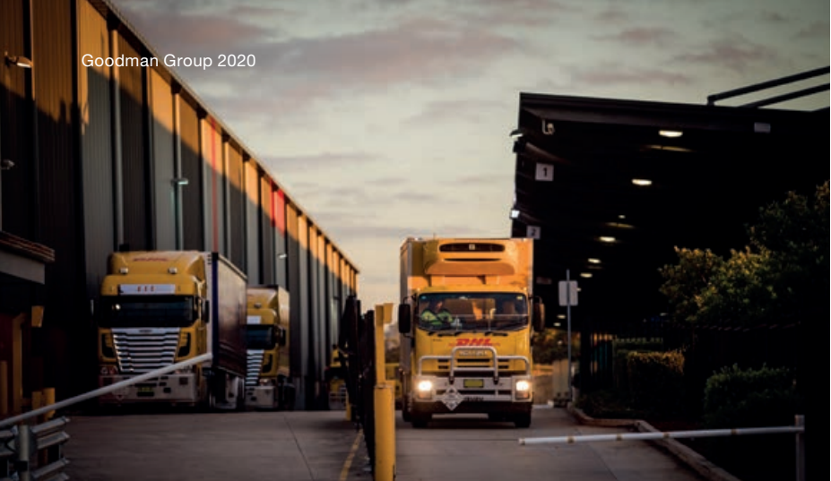
Oakdale Industrial Estate, Sydney, Australia.
