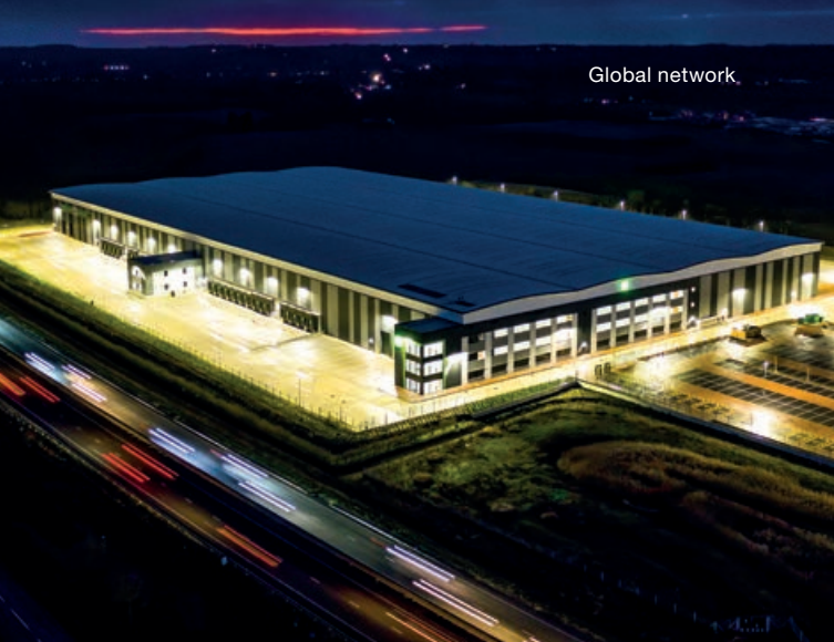
Bedford Commercial Park, Bedford, United Kingdom.
