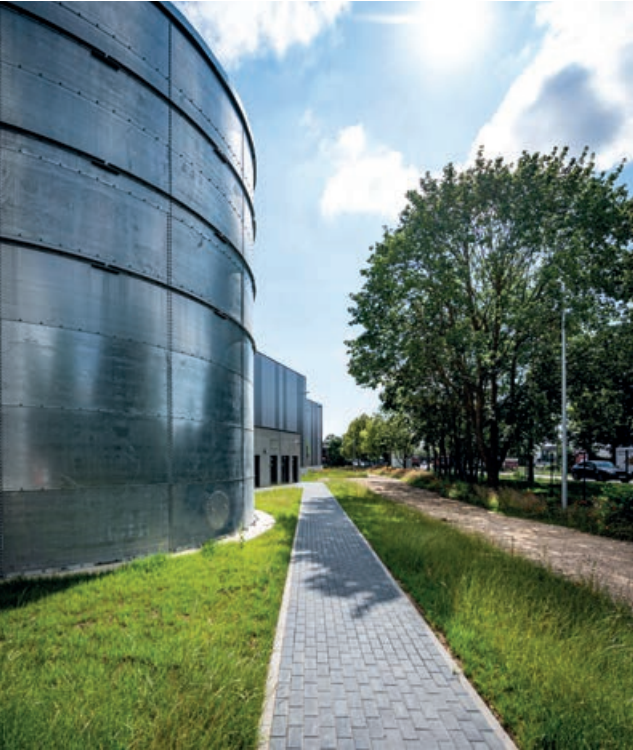
Regensburg I Logistics Centre, Regensburg, Germany.
