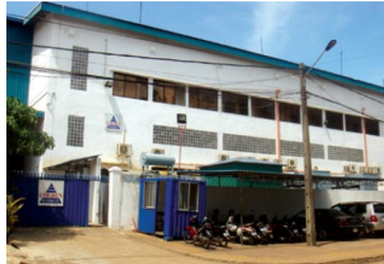
Sihanoukville Power Plant
