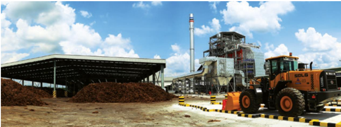
Figure 3. Maju Intan biomass power plant in Malaysia
