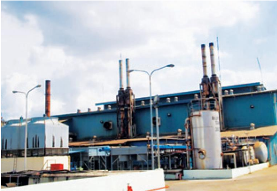
Phnom Penh Power Plant
