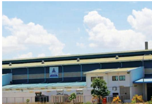
PPSEZ Power Plant
