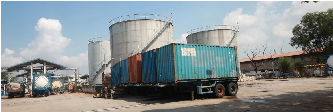
Figure 3: Sakra CIL chlor-alkali production plant/ Samulun CIL Logistic Base
