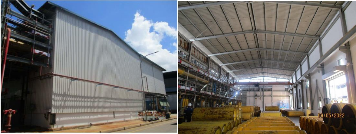
Figure 19: The chlorine filling area
