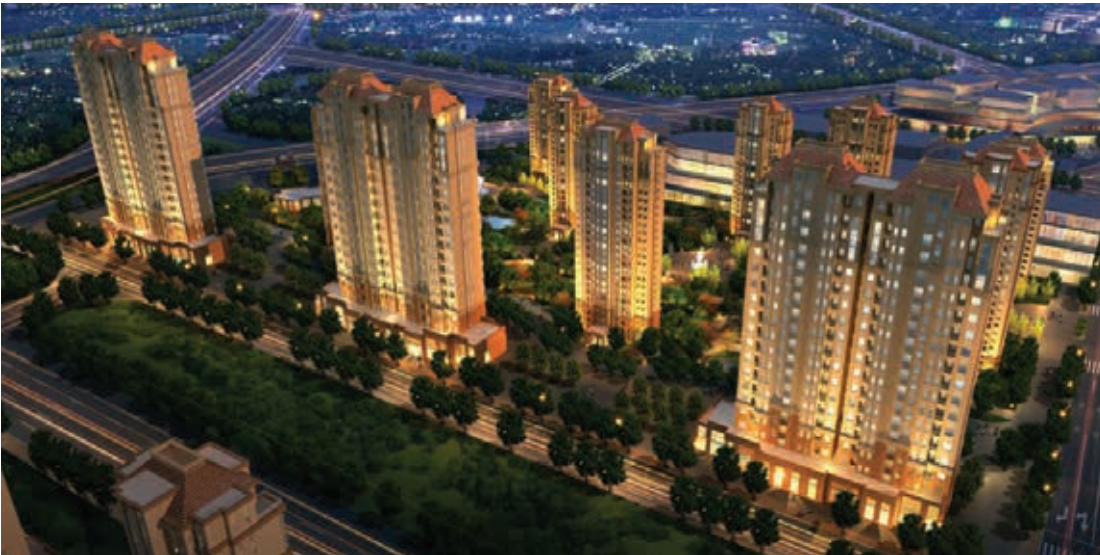
Tangshan Nanhu Eco City project
