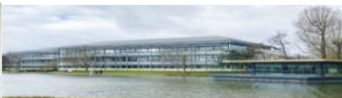
Building 1330 adjacent to Floating Pavilion
