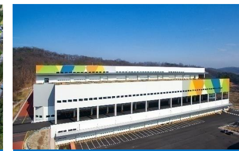
Mapletree Logistics Centre – Majang 3, South Korea
