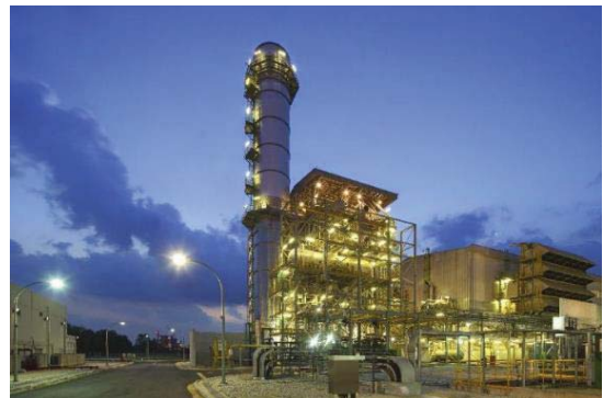
Keppel Merlimau Cogen (KMC) Plant, Singapore
