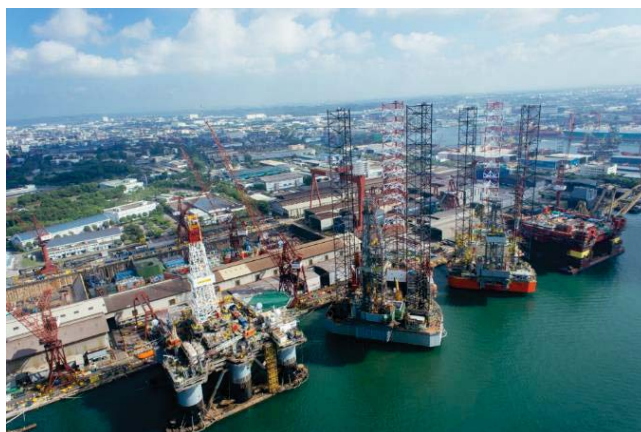
Keppel FELS, Singapore
