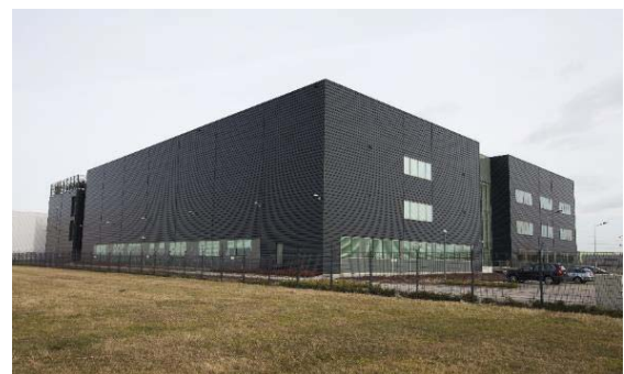
Almere Data Centre 2, the Netherlands
