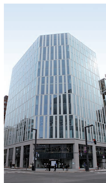
▲ Sapporo Fukokuseimei Koshiyama Building
