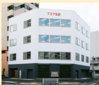
Koiwa Fukoku Seimei Building
