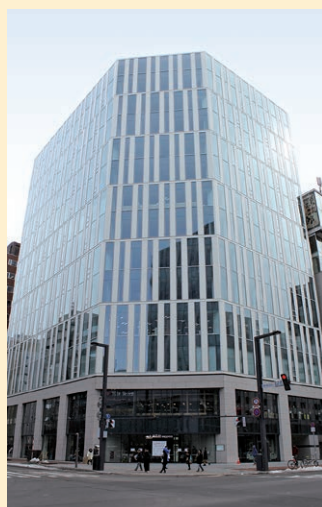
Sapporo Fukoku Seimei Koshiyama Building
