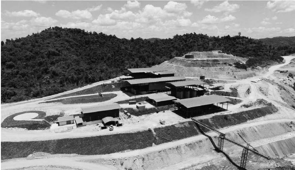
Figure 3.2 Sokor CIL plant and tailings facility – March 2019
