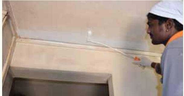
Cleaning & repainting works at Henderson
