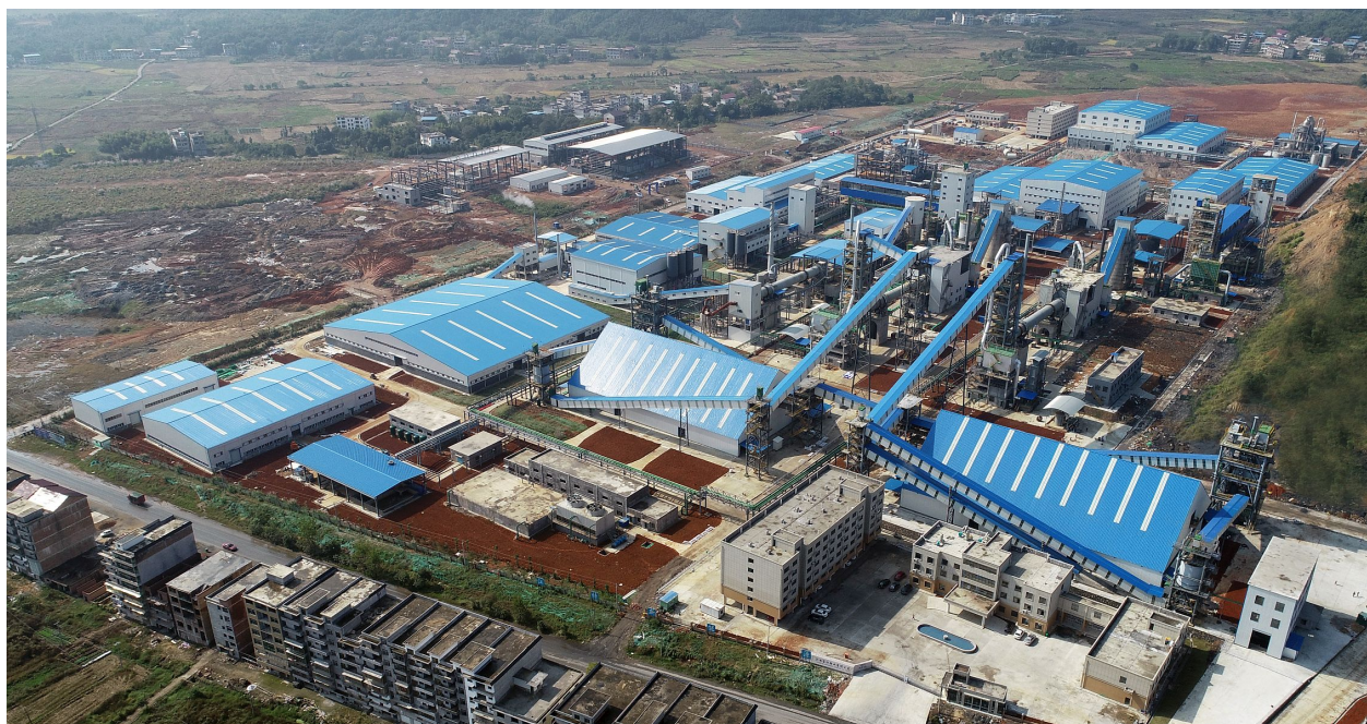
Figure 1 | Aerial view of Jiangte’s Yinli New Energy conversion facility which extends 800m by 350m
