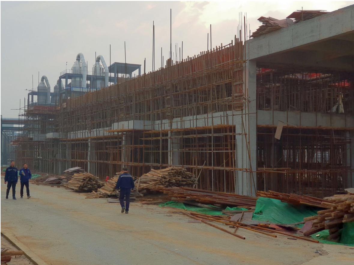
Figure 3 | Ongoing construction for hydroxide circuit in the foreground with existing leach circuit in the background at Jiangte's Yinli New Energy facility.
