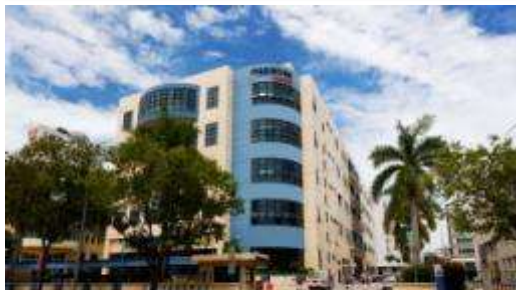
Light Industrial Buildings
