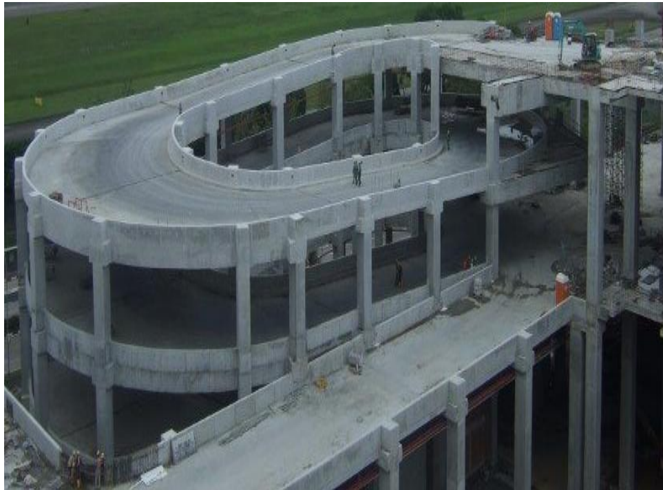
Overview of ramp
