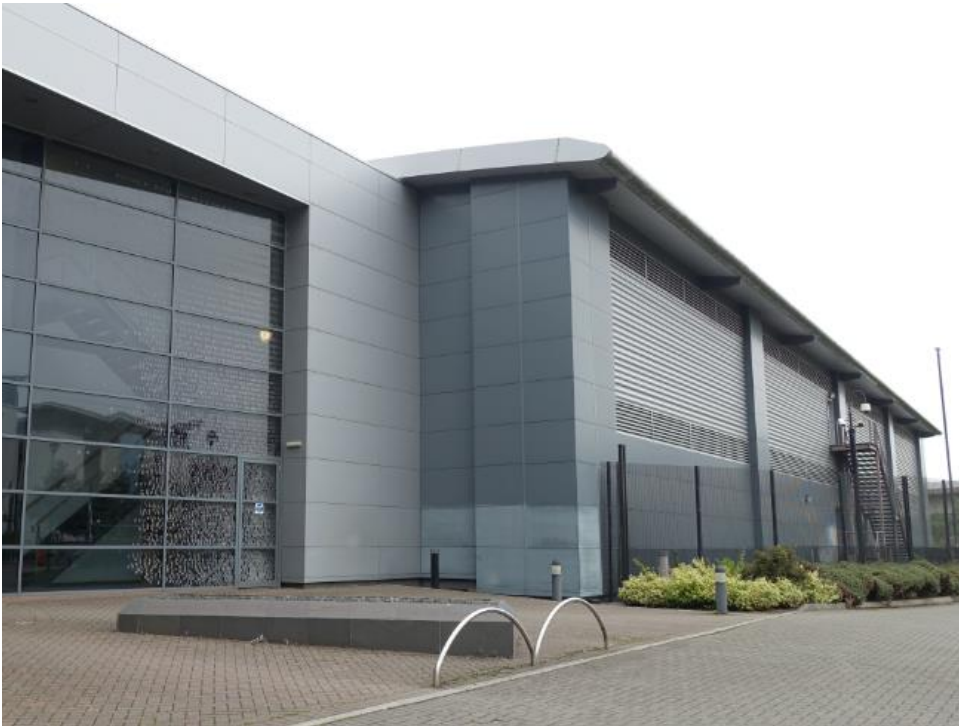
Data centre in Cardiff, United Kingdom
