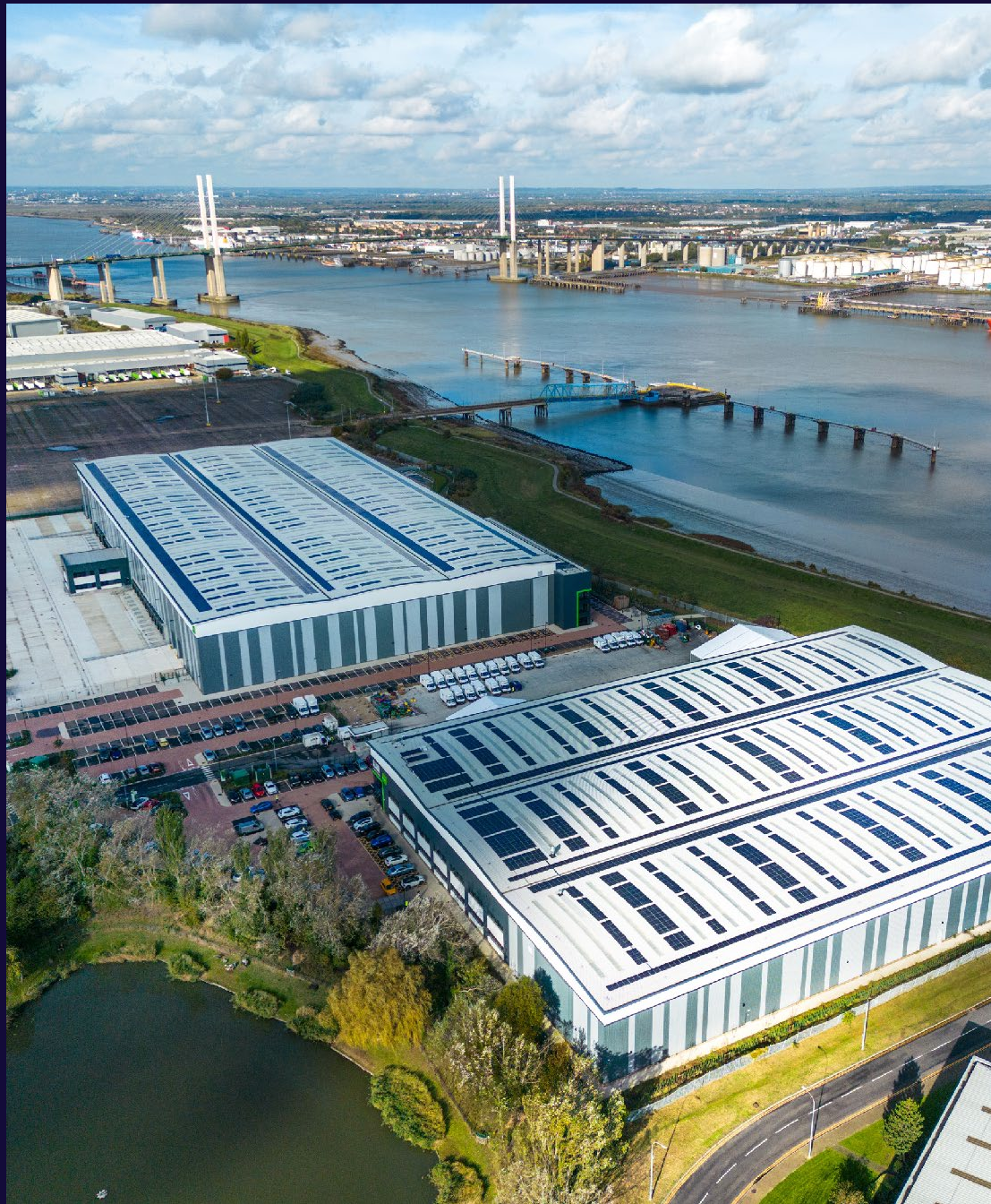
Crossways Commercial Park, London, UK
