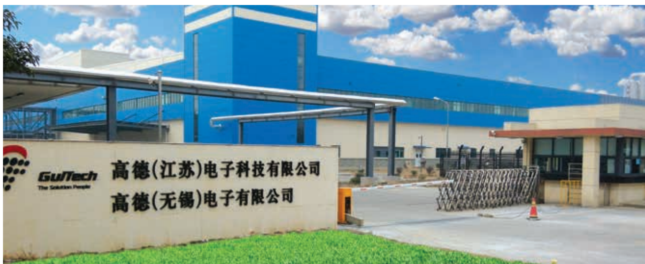
GulTech Jiangsu and Wuxi Factory Building, China
