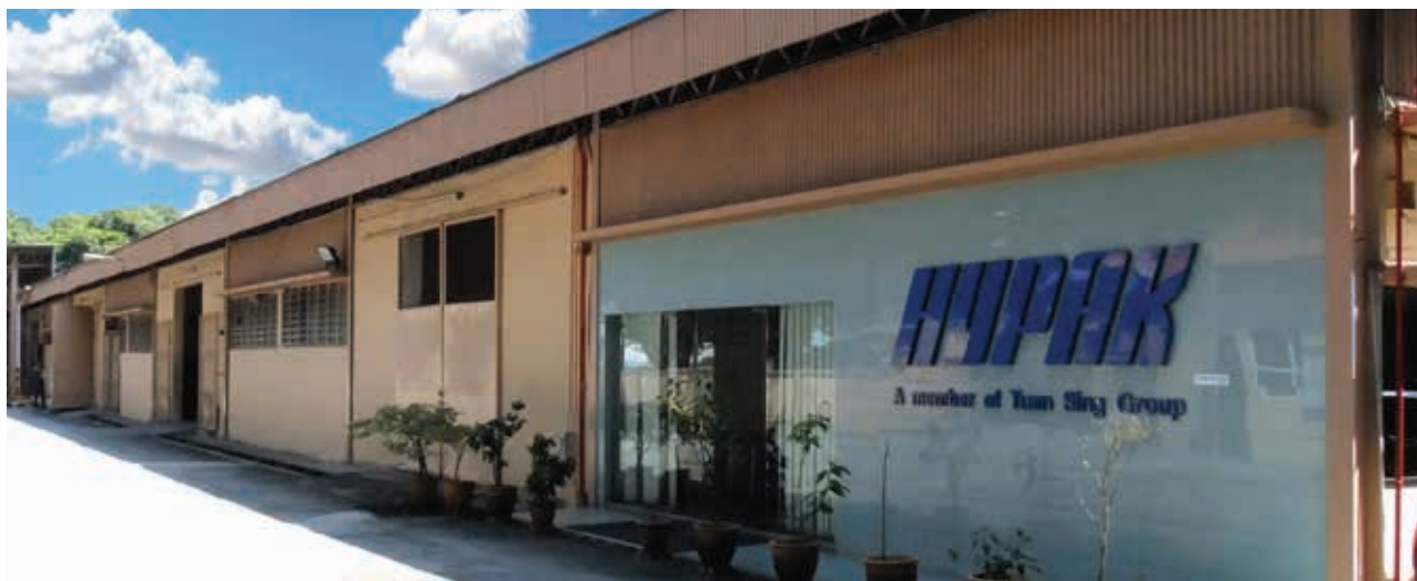
Hypak Factory Building, Malaysia
