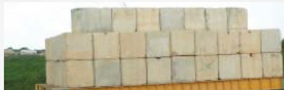
Concrete blocks used in static pile load test (Kentledge method). Source: BCA Build Smart Publication October 2013
