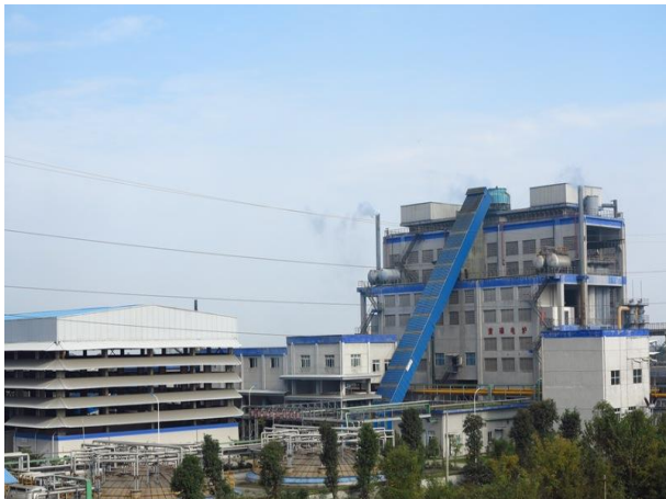
P4 factory / bulk storage
