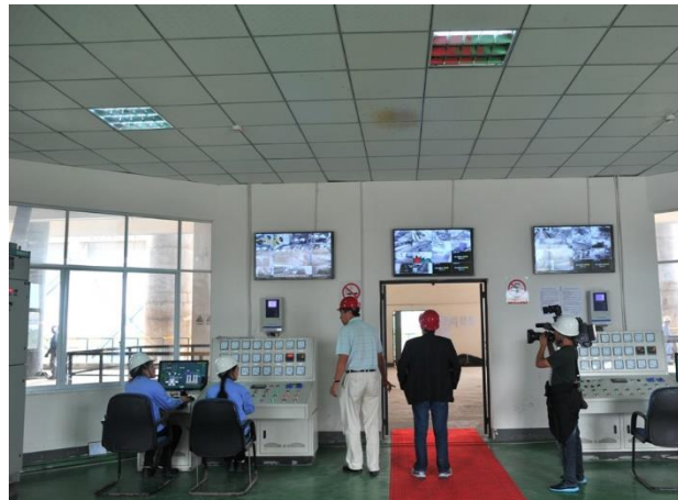
P4 factory control centre
