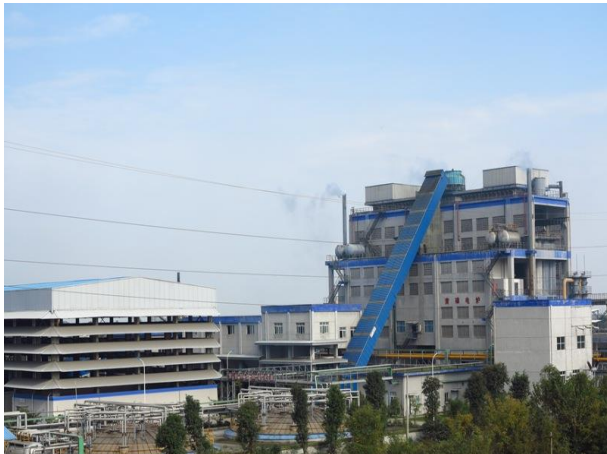
P4 factory / bulk storage
