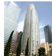
U.S. Bank Tower, Los Angeles (100% stake)
