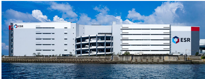
ESR Amagasaki Distribution Centre
