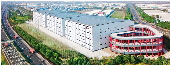
ESR Kunshan Huaqiao Park Phase III
