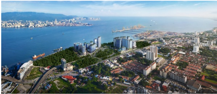
Aerial view of Straits City site
