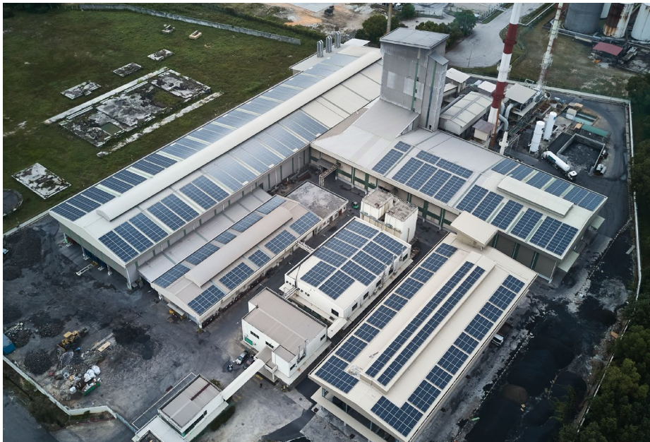
MSC's new smelting facility in Pulau Indah
