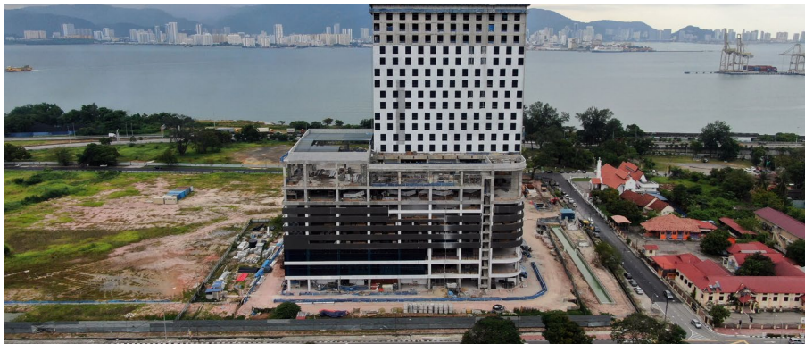
Construction of 4-star hotel in Straits City
