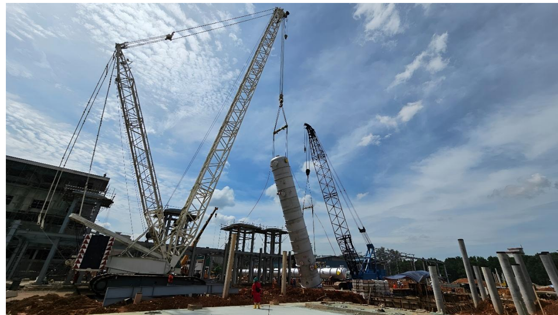
1,000T Crawler Crane
