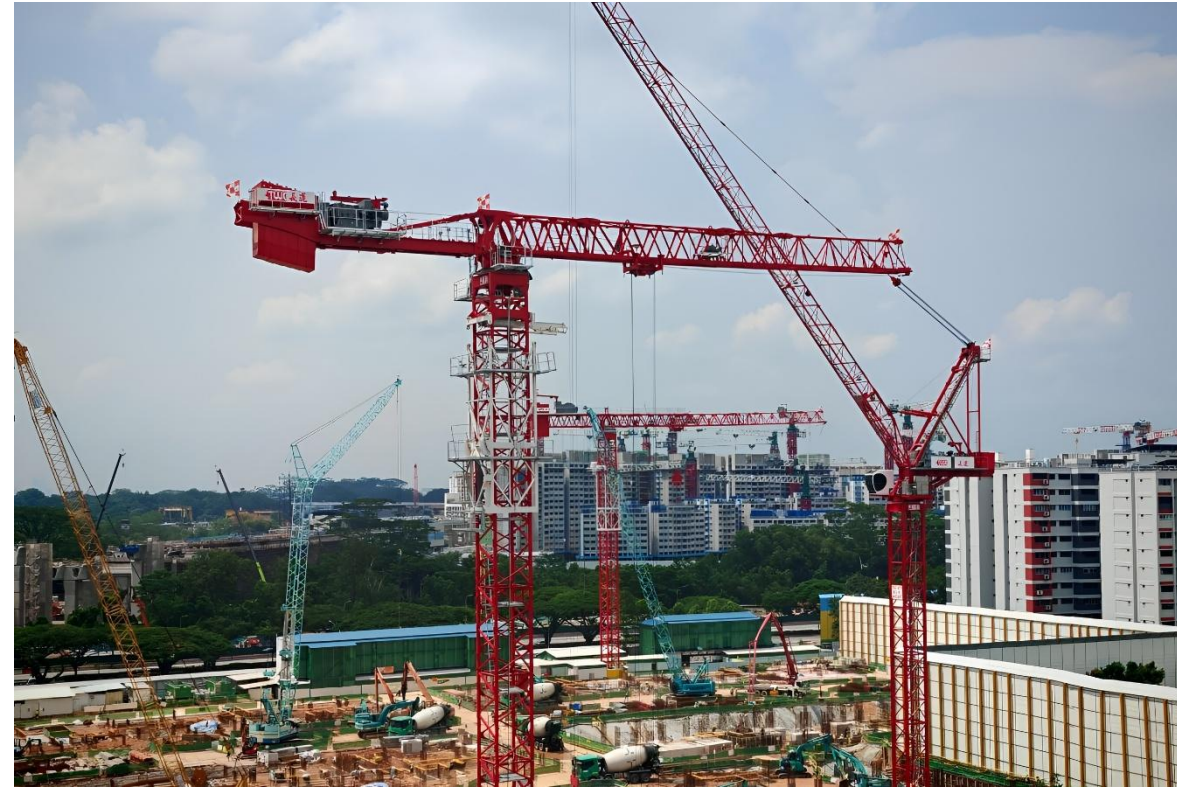
Potain Tower Cranes
