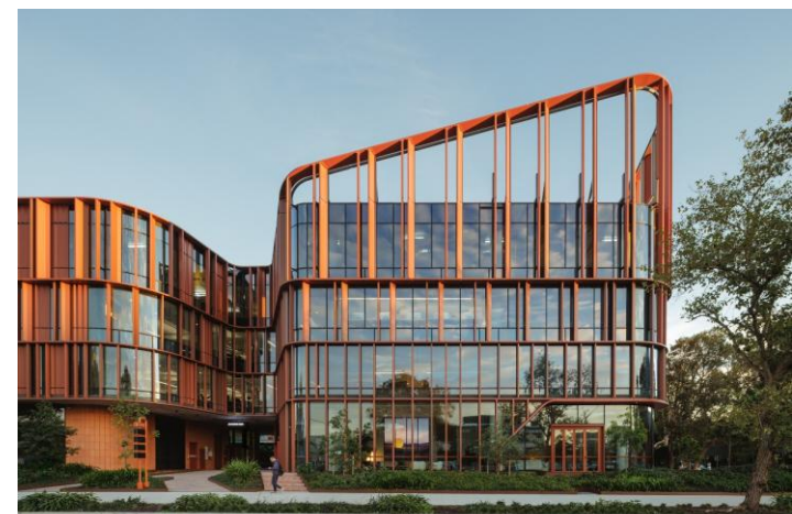
Pictured above is one the five assets that ACP II is providing private credit to, a campus-style Grade A office in Sydney, Australia
