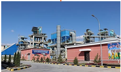
Mohir Grinding Station
