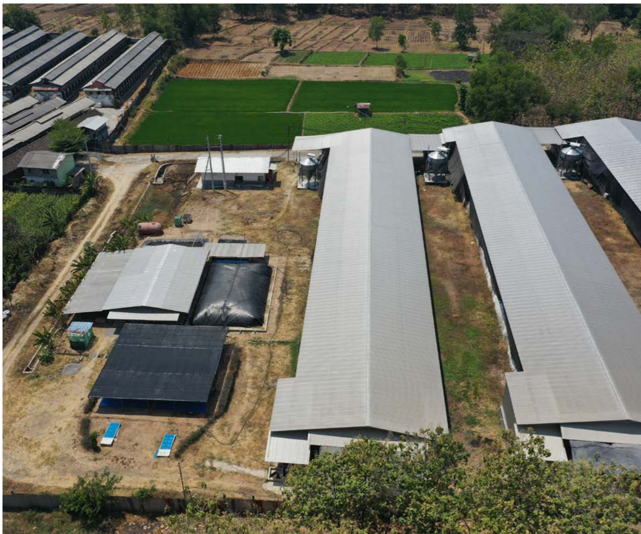
Biogas treatment facility in Commercial Farm unit
