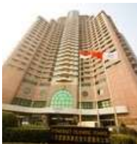
Somerset Olympic Tower Property Tianjin
