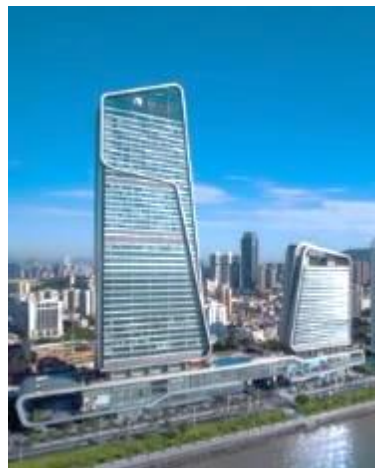
Yanlord Marina Centre, Zhuhai 仁恒滨海中心, 珠海 ▪ Office & Retail ▪ Total GFA: 42,974 sqm
