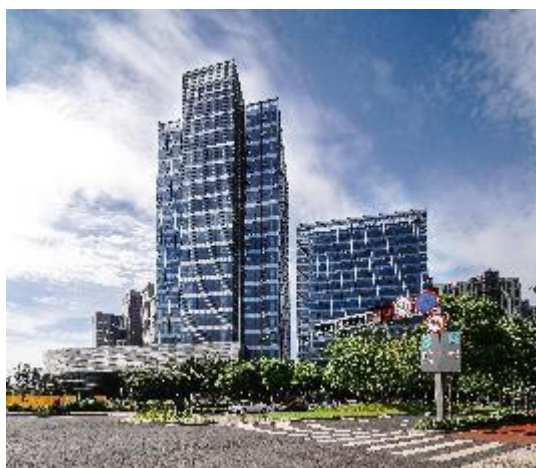
Yanlord Landmark, Nanjing 仁恒置地广场, 南京 ▪ Office & Retail ▪ Retail: 23,420 sqm ▪ Office: 83,744 sqm
