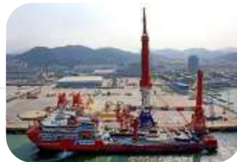
Installation of Huisman crane
