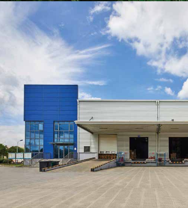
Initiated the installation of solar panels on the roof of Kunshan Bacheng Logistics Park
