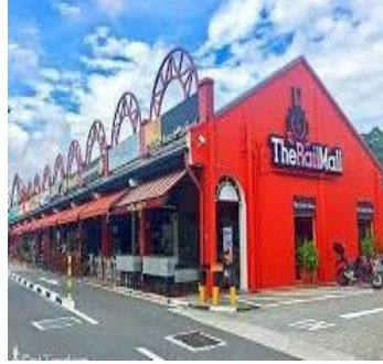
The Rail Mall S$63.8m
