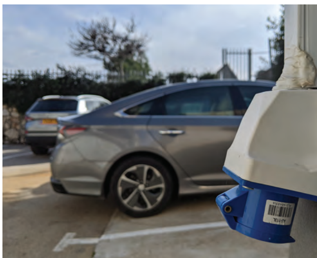
Charging station for electric at our headquarters in Israel
