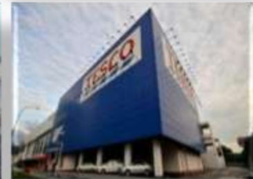
TESCO Building Penang
