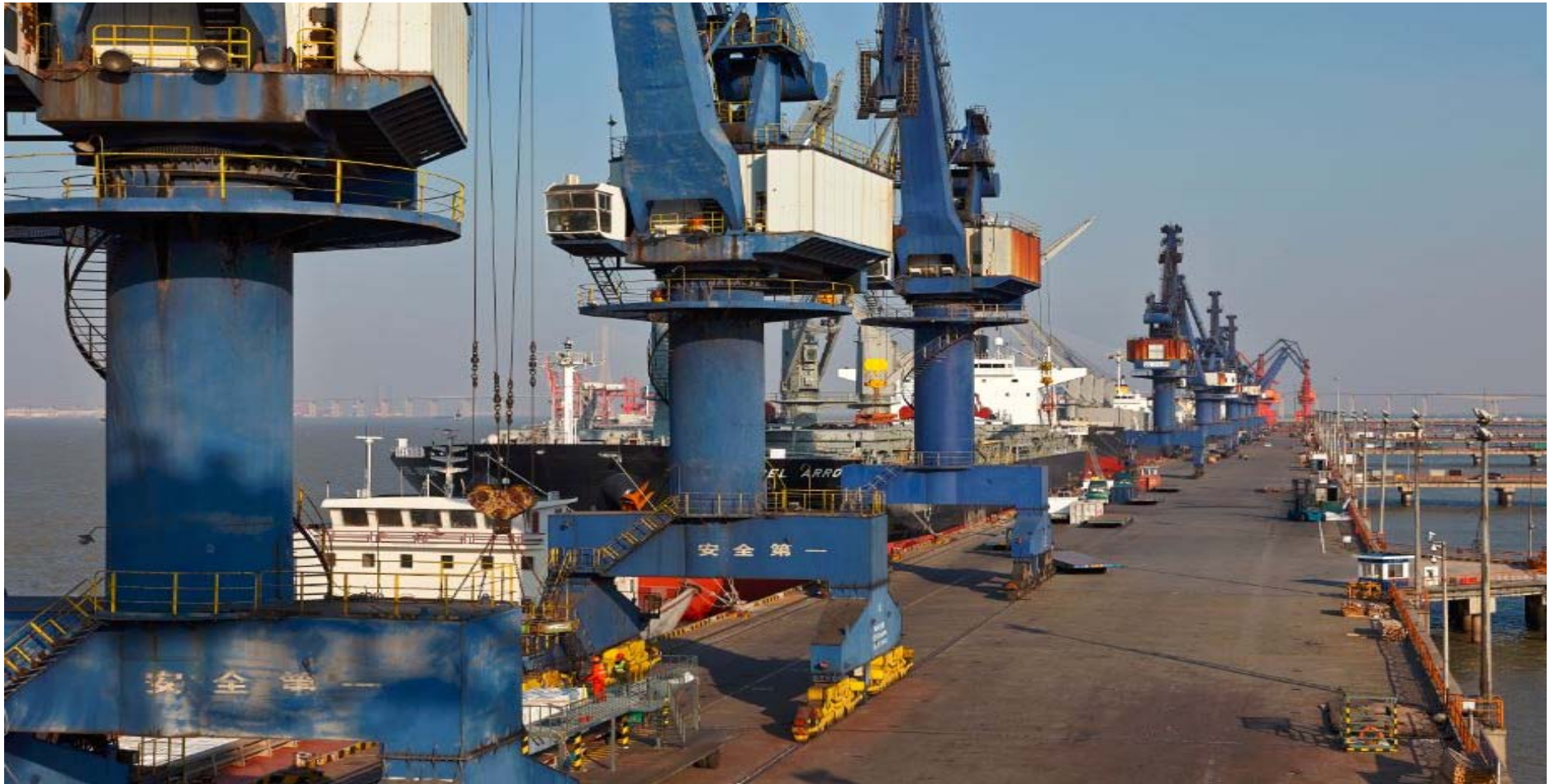
Multi-purpose facilities for bulk and containerised cargoes
