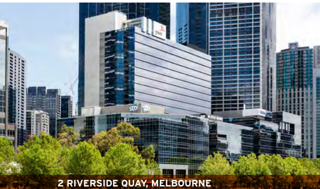
2 RIVERSIDE QUAY, MELBOURNE
