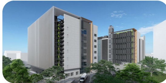
Keppel Data Centre Campus, Singapore
