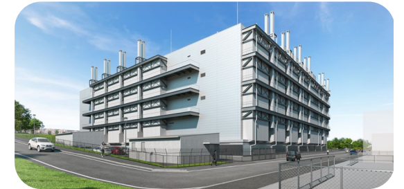
Western Tokyo Data Centre
