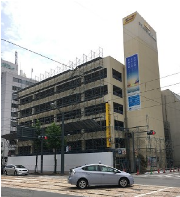
Original building at the site before demolition
