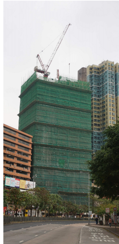
Site currently under construction
