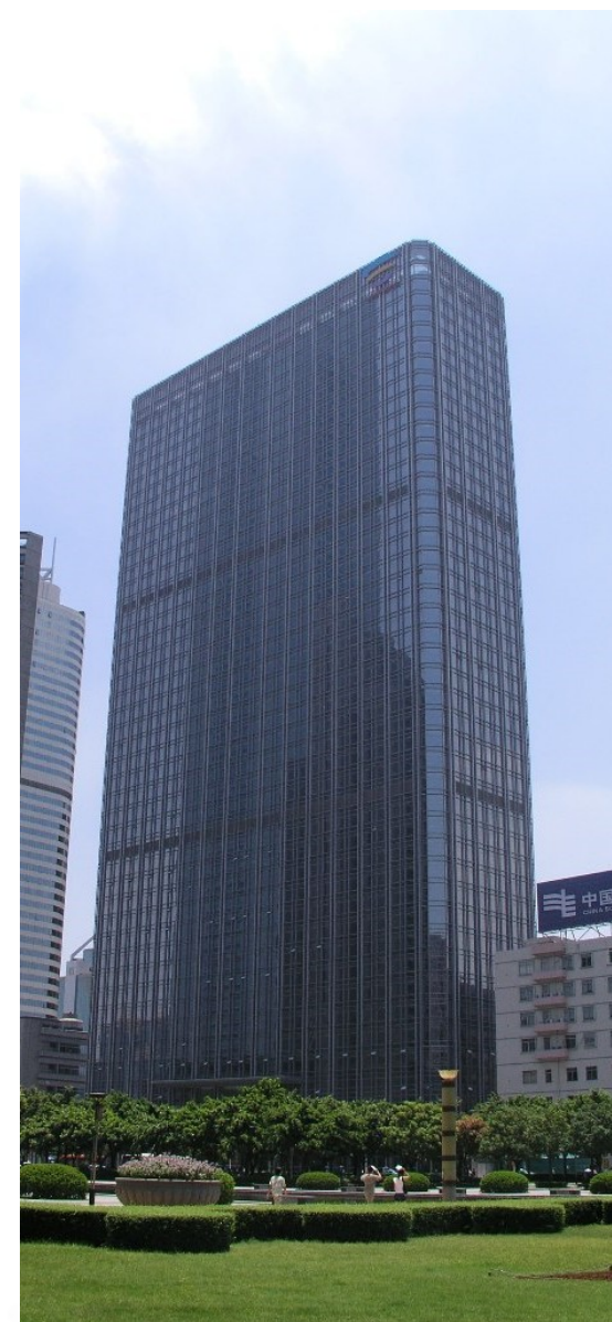
China Shine Plaza in Guangzhou, China
