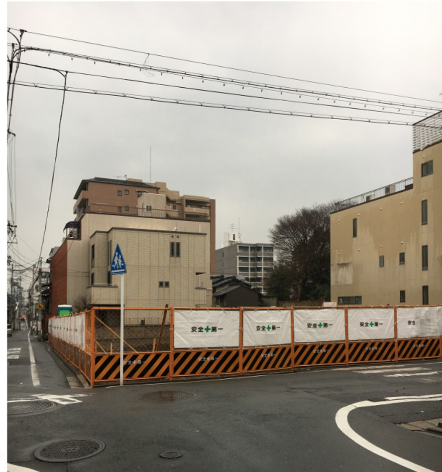
Existing site after demolition of original building
