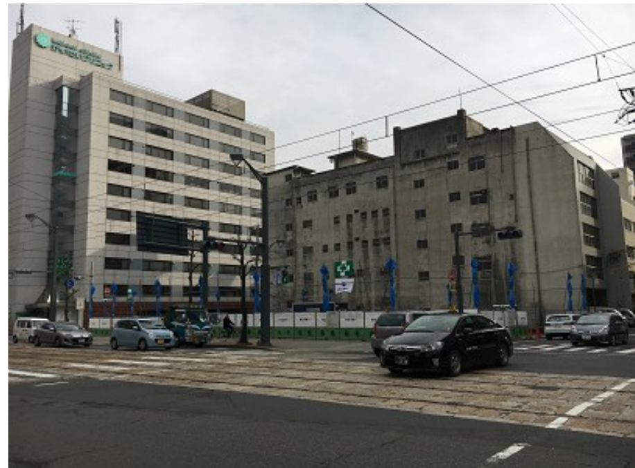
Existing site after demolition of original building
