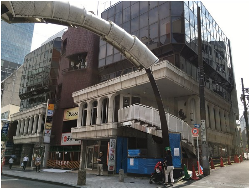
Original building at the site before demolition
