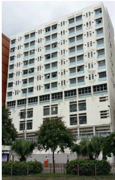
Original building on the land before demolition
