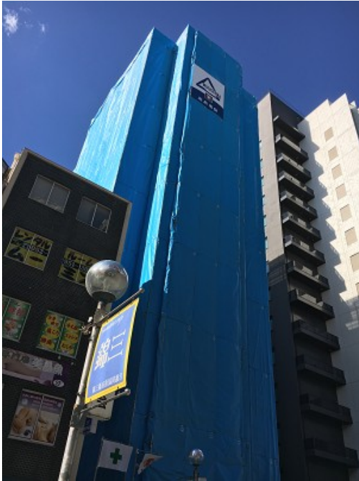
Current construction progress
