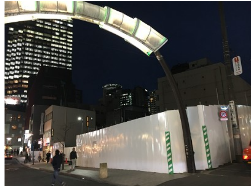
Existing site after demolition of original building
