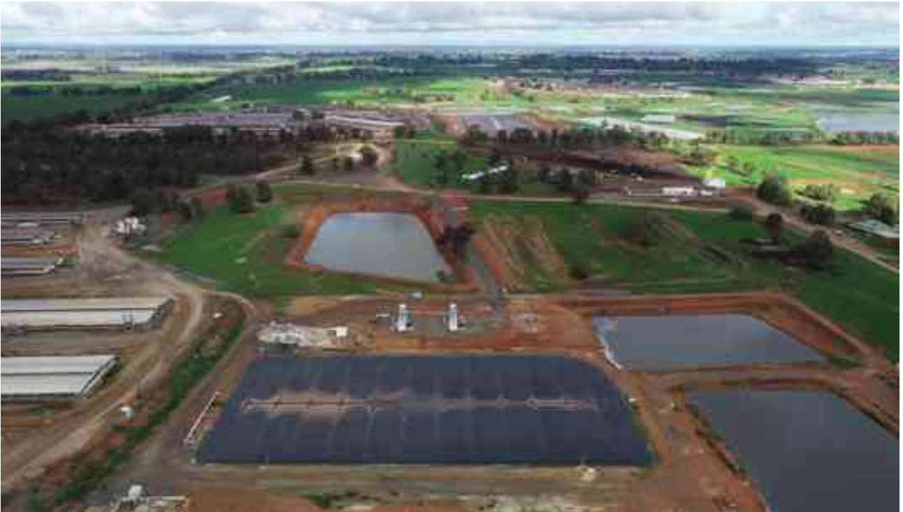
Rivalea's biogas collection facility at Corowa, NSW.
