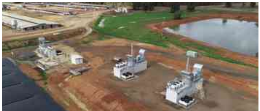
Rivalea's biogas electricity generators supplied from captured methane, Corowa, NSW.
