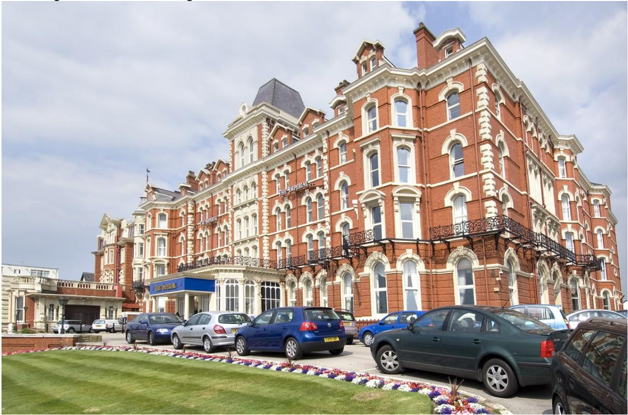
Front façade of the hotel building
