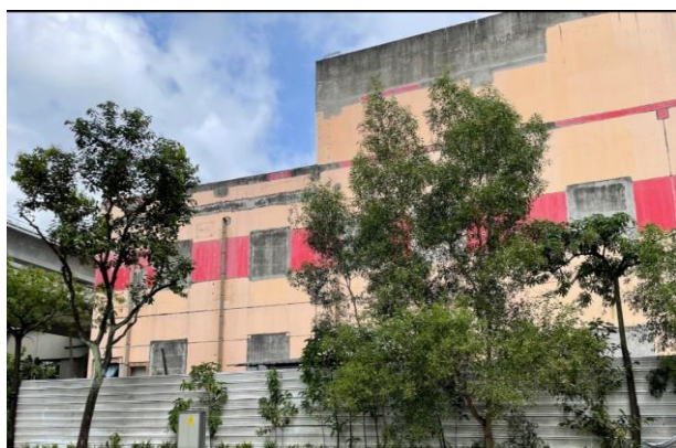
Pre-AEI property at 1 Tuas Avenue 4
