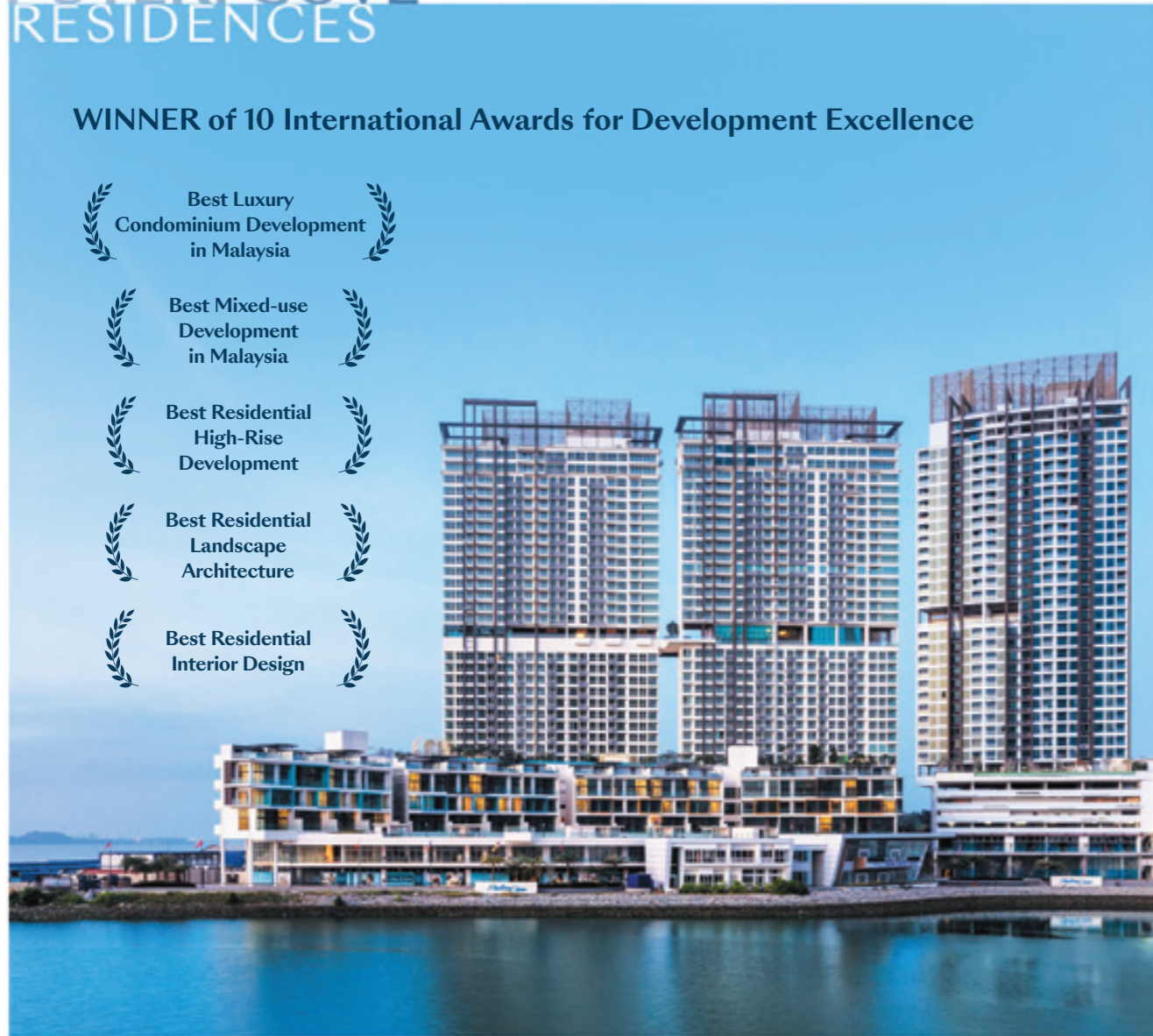
Puteri Cove Residences successfully attained its Certificate of Completion and Compliance in 2018. The multiple award-winning luxury mixed-use development is widely recognised as one of the most successful projects in Iskandar Puteri with buyers from more than 28 countries.
