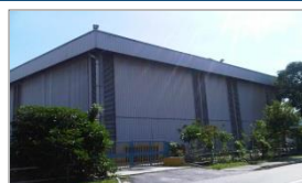
3 Kim Heng Warehouse 4 Penjuru Lane
