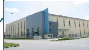
10 APC Distrihub 6 Changi North Way
