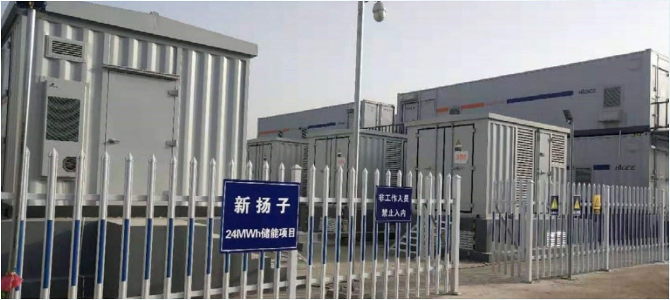
As part of the Group's efforts for sustainability, a power storage station was set up, utilizing lithium batteries to support and reduce electricity consumption.
