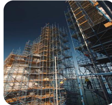
CBH Shiploader Refurbishment
